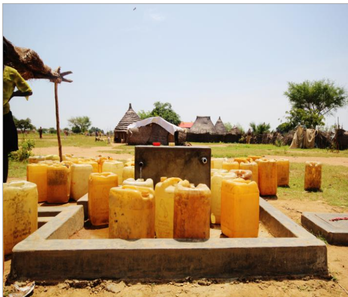
Figure 11: Queue of jerry cans forming at Wanjok, because of low water pressure
