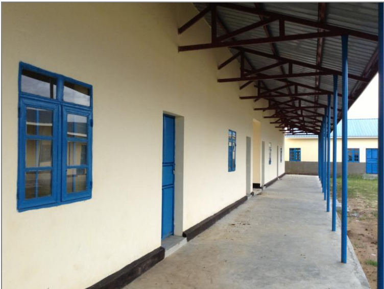
Figure 14: School dormitories constructed by IOM in Mayen Abun
