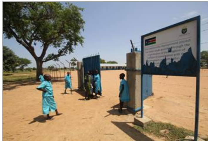
Figure 10: School fence and gate at Malualkon School
