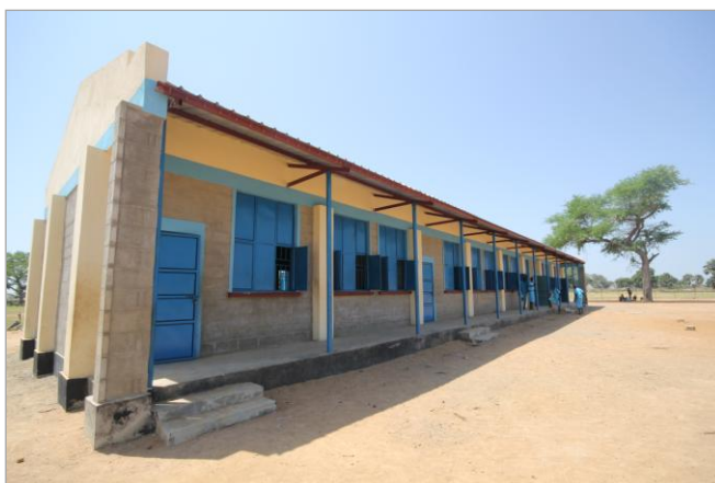
Figure 9: Newly constructed school building at Malualkon School
