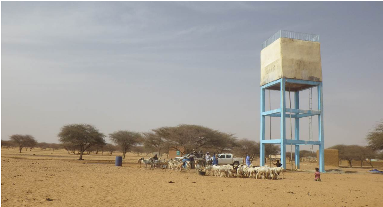
Figure 3: Water tower in the village of Sissakou
