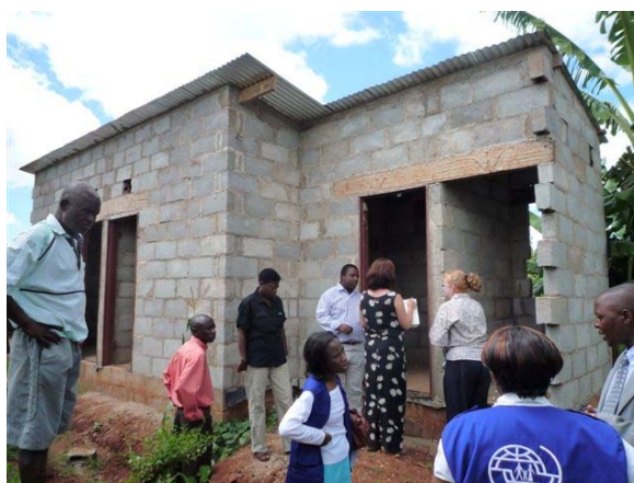
'Finished' transitional shelter in Hatcliffe (Photo: P. Holdsworth 2009)
